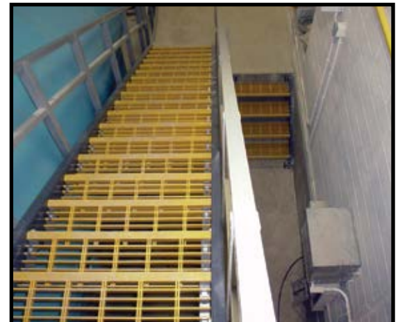
The stairway above utilizes Fibertred molded stair treads to provide tank access at a pumping station.
